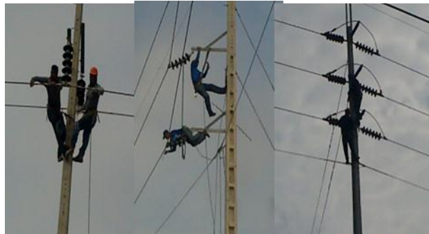
Figure 4. Electrical workers cleaning and maintaining networks
