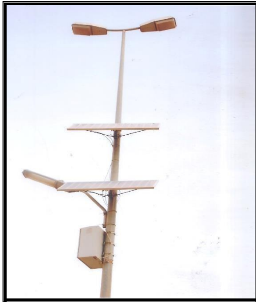
Picture 1 Solar cells used for lighting in one of the governorate's streets The photo was taken on April 30, 2020
