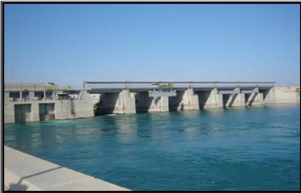
Picture 4 Al-Kufa Barrage in Najaf Governorate The photo was taken on 4/28/2020
