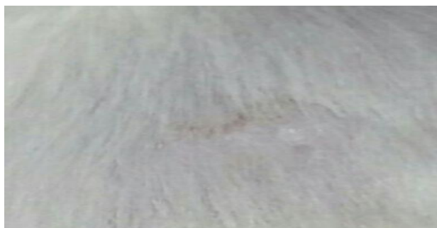
Figure 12. Day 10 (After removal of plaster the scar was observed)
