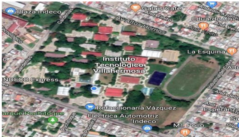
Figure 1. Aerial view of ITVH and Building Z
