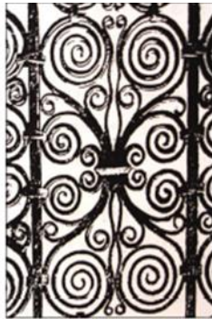
Figure 2. Assembling the modules using ligatures - Puyi Cathedral
