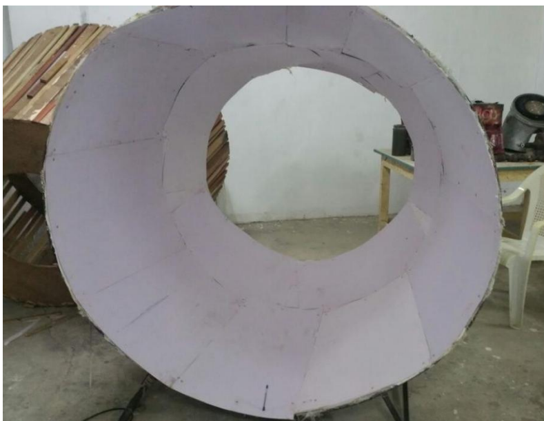
Fig 3.7 Preparation Of Duct
