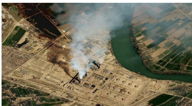
Figure 1.3: Zubaidiya power station from an aerial view
