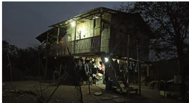
Figure 4. Illuminated housing at night
