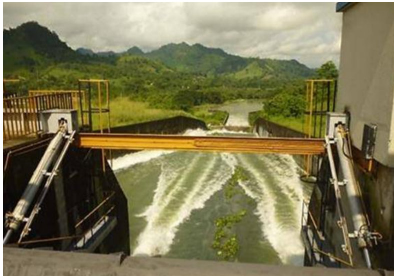
Figure 2. Gate of the La Esperanza Dam
