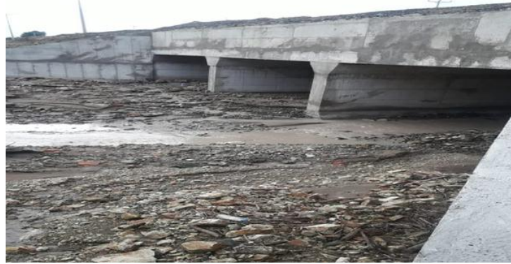
Figure 2. Triaduct studied on March 7, 2019
