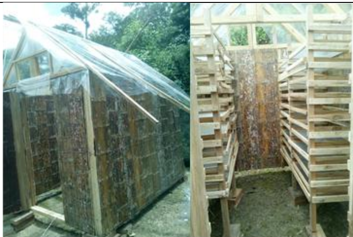
Figure 4. Solar grain dryer built with cane Guadua
