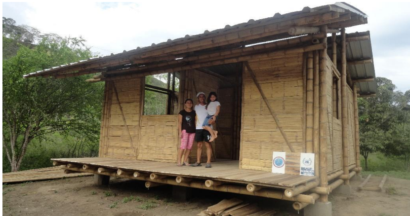
Figure 4. Emerging housing completed
