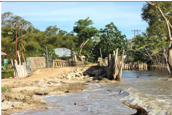
Figure 5. Tidal floods that have risen to the body of the road around the Ndalir beach (Batbual, 2014)
